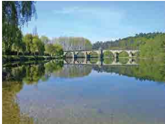
Bridge over river Lima
