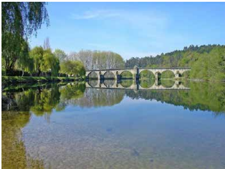
Bridge over river Lima
